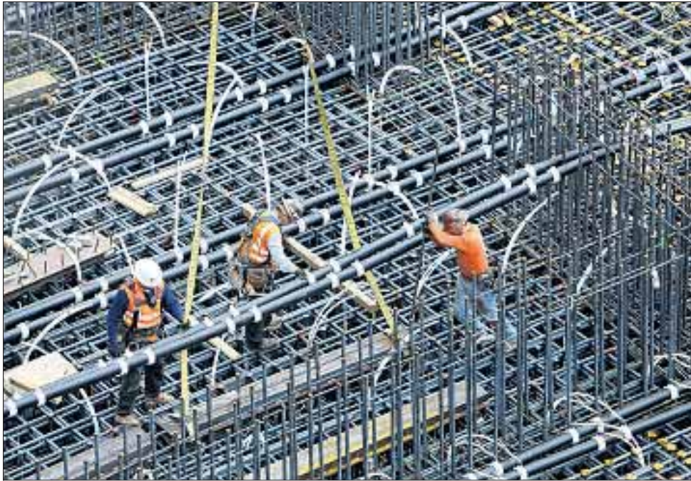
WORKERS POSITION pipes into place while standing above an 18-foot hole that will be filled with concrete to form the foundation for the project.
