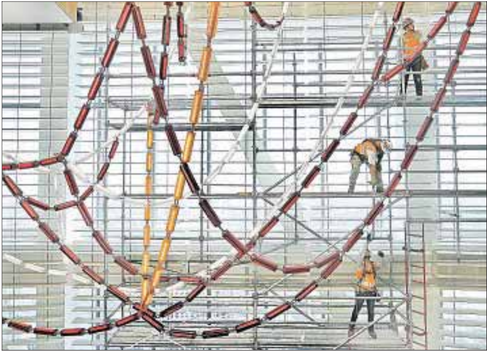
SCAFFOLDING is erected to install louvers and a three-story-high chandelier.
