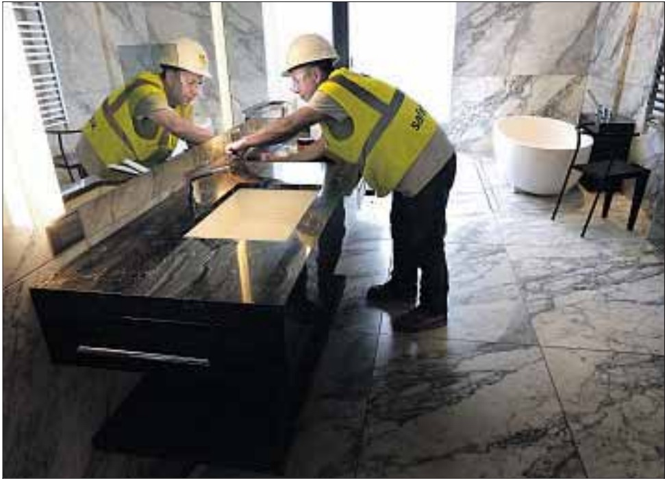
A MARBLE countertop is installed in the master bath of the Presidential Suite.
