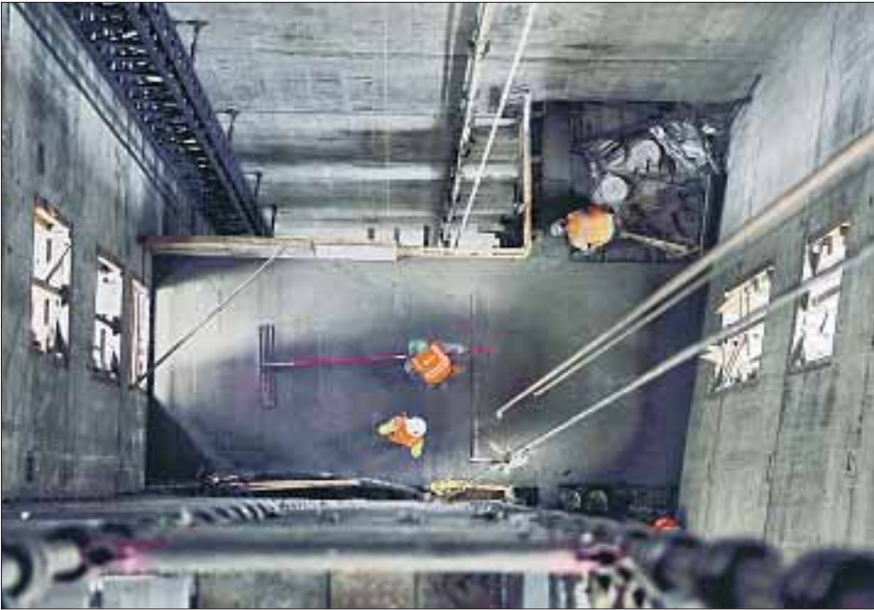
CEMENT FINISHER Jaime Velasquez, center, smooths out a concrete deck after it is poured on the 9th floor of the concrete core of the Wilshire Grand.
