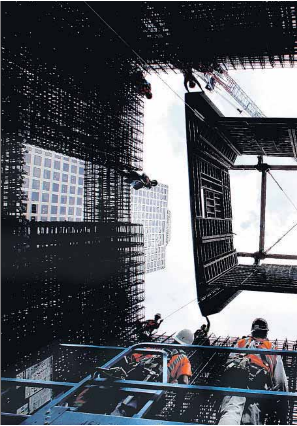
CONSTRUCTION WORKERS guide a jumping wall form system into place as it is lowered into posi-
