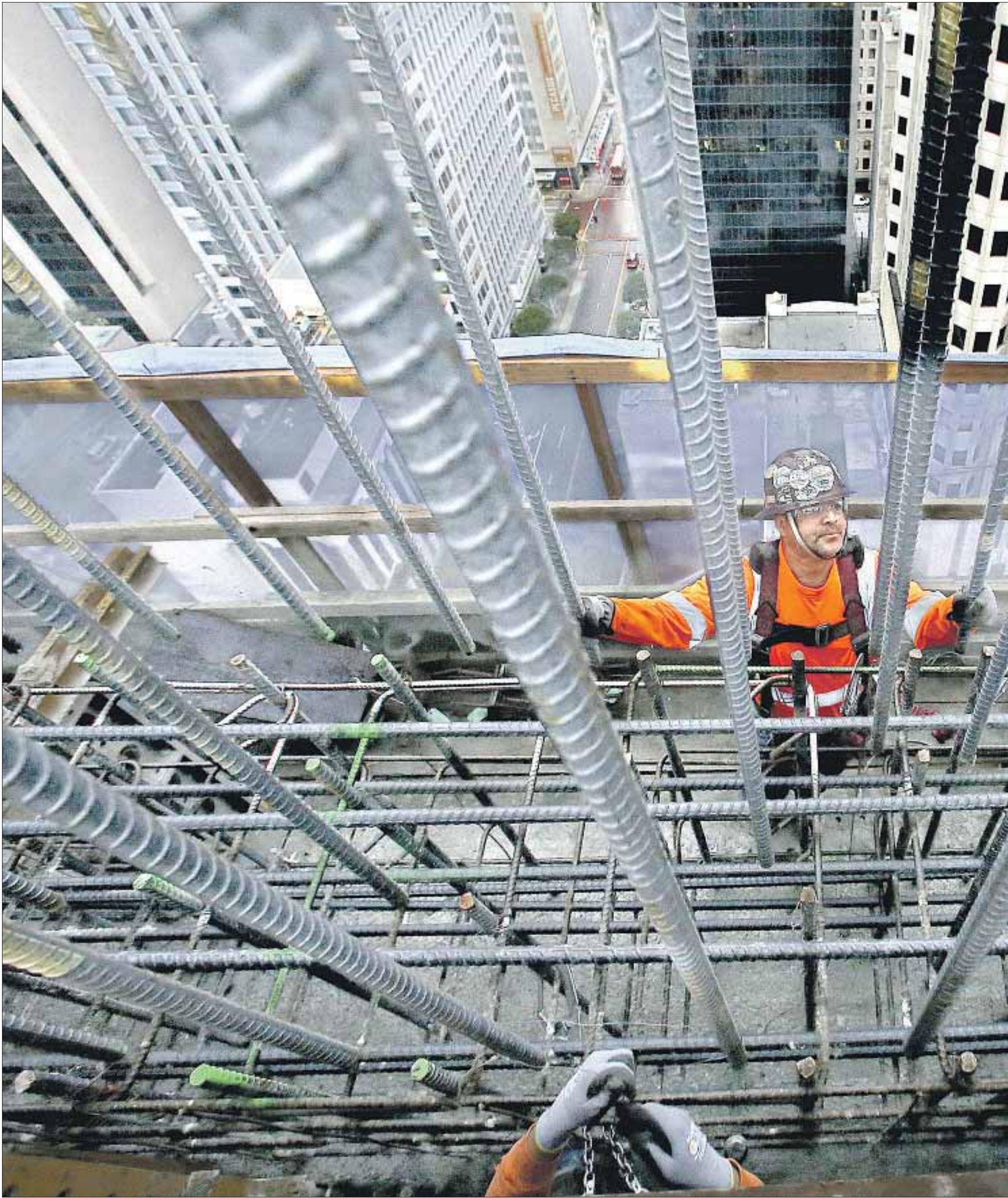
IRON WORKER Javier Jimenez guides a rebar wall into position as it hangs from a crane above. Rebar, which provides strength to concrete that would otherwise crack
